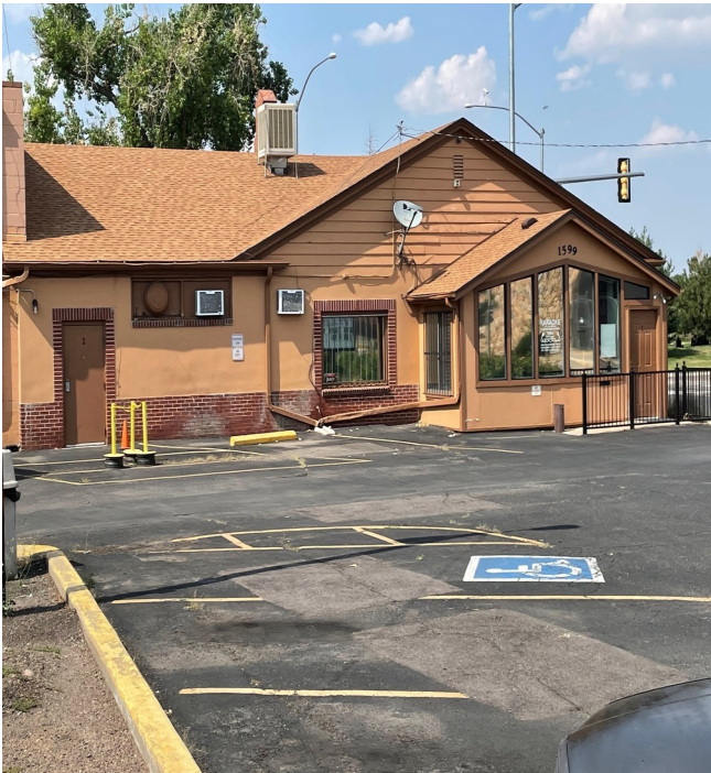
Front of the Chapter 3 Building.
